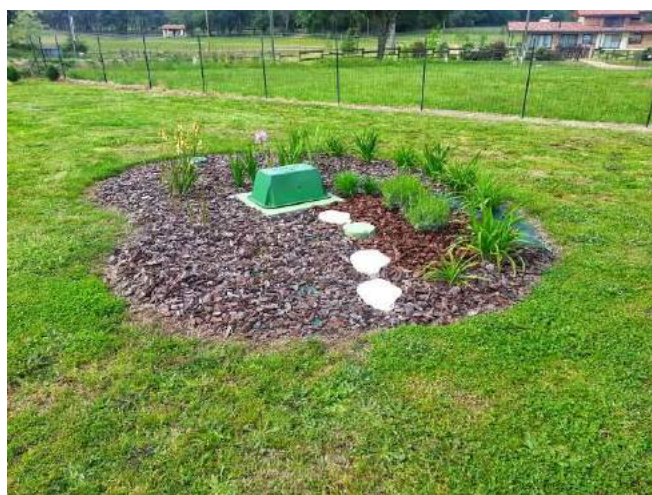
Micro-station Tricel Novo FR6/4000 installée
