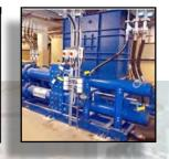
The Saxlund Solids Pump has been reliably conveying all types of sludge cake for many years. Transporting sludge cake in closed systems keeps it separate from its surroundings and the environment.
