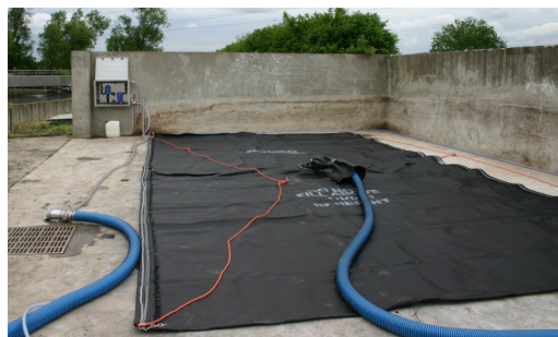
Installation Station Longperrier (77)
