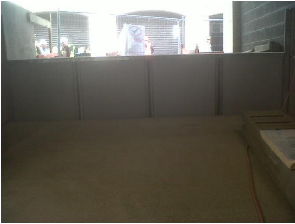
Fig 9. 2012: Jersey - USA. Protection d'un parking souterrain.
