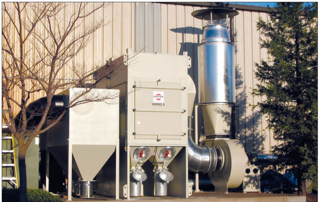
VARIO 6 eco with chip preseparator and fan including exhaust silencer
