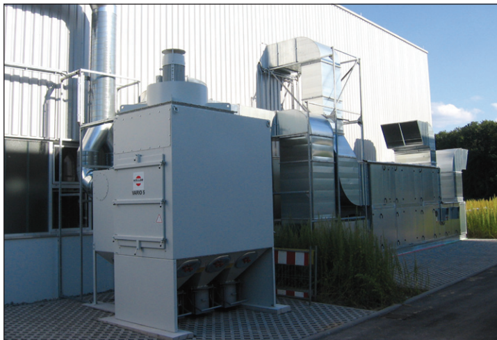
VARIO 5 eco with spark preseparator and heat recovery system
