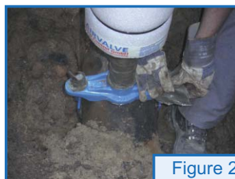
Figure 2 Application de la protection anti-corrosion de la connexion.
