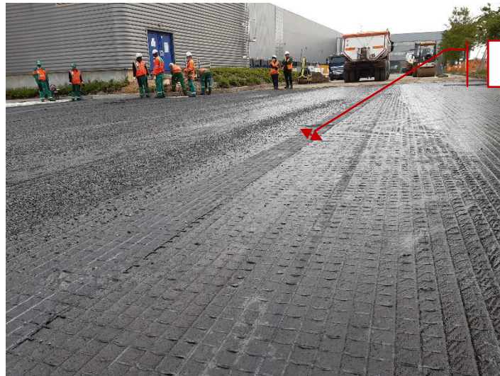
FIGURE 14 : RECOUVREMENT COTE-A-COTE
