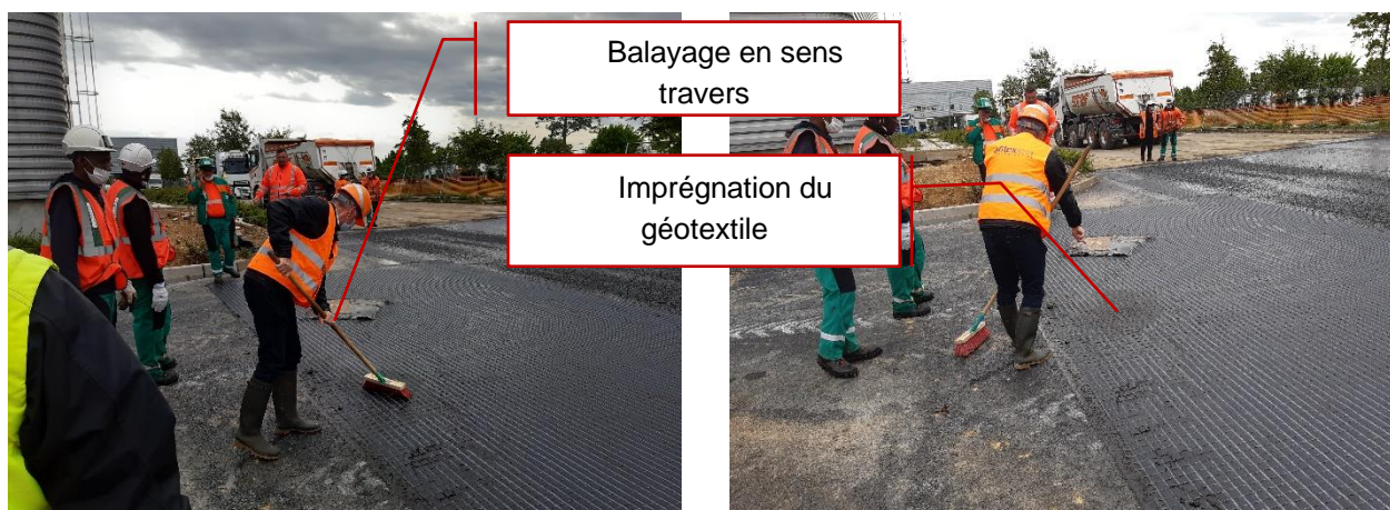
FIGURE 11 : BALAYAGE ET IMPREGNATION
